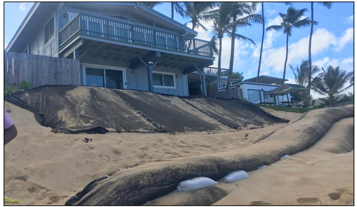
Unauthorized sand burritos installed below Gary and Cynthia Stanley's Sunset Beach property.
